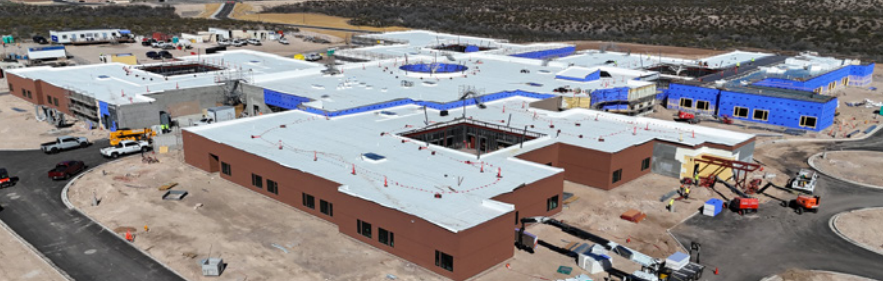
CONSTRUCTION SITE OF THE SADIE KNIFFIN LONG TERM CARE AND SKILLED NURSING FACILITY
