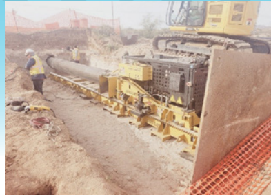
CONTRACTOR PERFORMS "JACK AND BORE" BENEATH HIGHWAY 70. THIS IS A HORIZONTAL AUGER BORING METHOD WHERE A 24-INCH STEEL CONDUIT PIPE IS ADVANCED BENEATH THE HIGHWAY FOR INSTALLING A PIPELINE CROSSING WITH MINIMAL TRAFFIC DISRUPTION.
