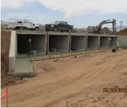
NEW CONCRETE BRIDGE INSTALLED ON ROUTE SIX TO ACCOMMODATE FOR POTENTIAL FLOODING
