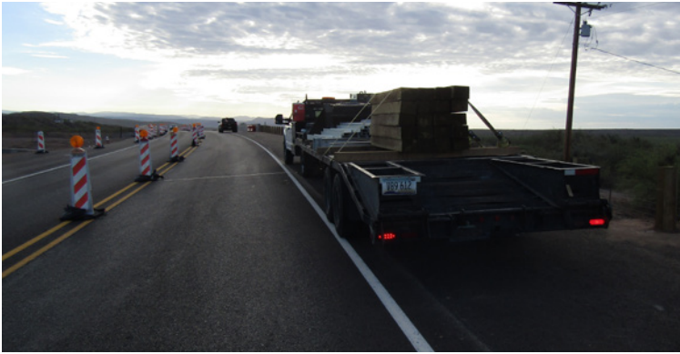
AREA ON ROUTE SIX WHERE CONSTRUCTION TOOK PLACE FOR BRIDGE
