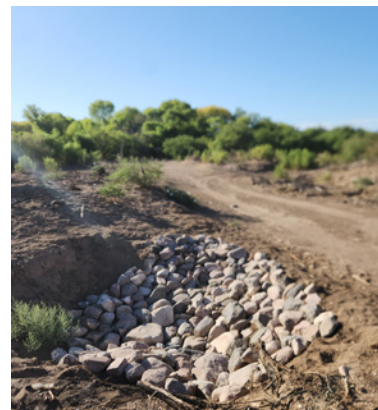
ROCK WORK SUPPORTS ROADS, REDUCES EROSION, AND CREATES EPHEMERAL POOLS
