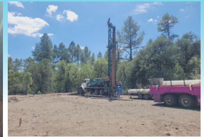
CONTRACTOR DRILLING OF A NEW STOCK WATER WELL IN RED BOX CANYON ALONG CAMP CREEK.
