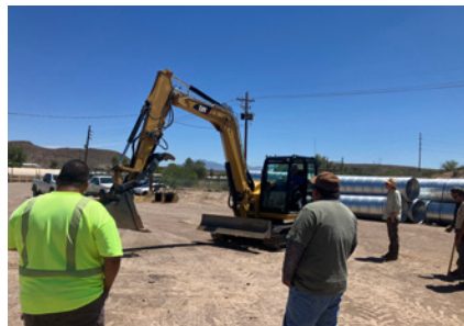
EXCAVATORS ENABLE PRECISE MATERIAL PLACEMENT FOR ROAD AND HABITAT RESTORATION
