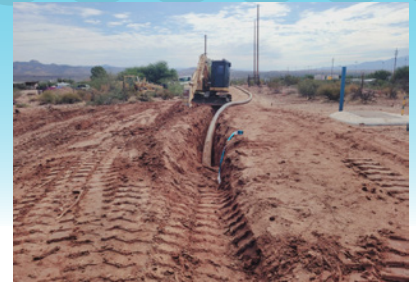
CONTRACTOR INSTALLS A NEW PIPELINE FROM THE NEW WATER TANK SITE TO CONNECT TO THE APACHE BURGER WELL ABOUT HALF A MILE AWAY. THIS PORTION OF THE PIPELINE IS ALONG THE NORTH SIDE HIGHWAY 70. A TRENCH IS DUG, THE WATER LINE IS INSTALLED, AND BACKFILL MATERIAL IS INSTALLED AND COMPACTED.
