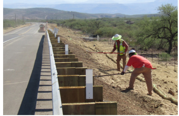
CLEANING FOR INSTALLATION OF NEW GUARD RAILS ALONG ROUTE SIX
