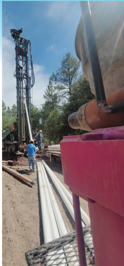
CONTRACTOR INSTALLING THE WELL CASING AT THE NEW RED BOX CANYON STOCKWATER WELL.
