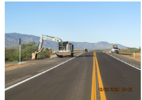
ADDING FRESH NEW STRIPES TO THE ROAD
