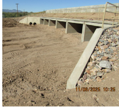
NEW CONCRETE BRIDGE INSTALLED ON ROUTE SIX TO ACCOMMODATE FOR POTENTIAL FLOODING
