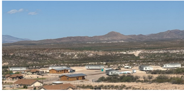
INDIAN HILLS HOUSING DEVELOPMENT IN CONSTRUCTION PHASE, SAN CARLOS, AZ
