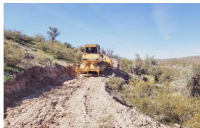
CONTRACTOR GRADING THE ACCESS ROAD TO THE NEW DRIPPING SPRINGS WATER TANK SITE.
