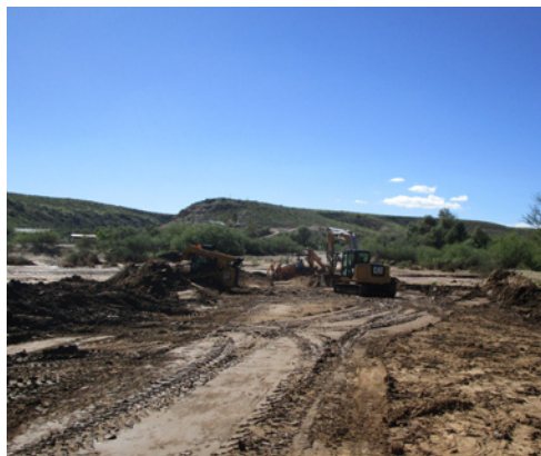
EQUIPMENT OPERATORS WORKING TOGETHER TO REPAIR FLOOD DAMAGE
