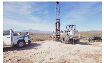
CONTRACTOR DRILLING AND COLLECTING SAMPLES FOR GEOTECHNICAL ANALYSIS AT THE NEW DRIPPING SPRINGS WATER TANK SITE. SEVERAL BORINGS WERE DRILLED AND TESTED TO ASSESS THE SOIL CHARACTERISTICS TO PROPERLY DESIGN STRUCTURAL FOOTINGS FOR THE TANK, THE PIPELINE BACKFILL MATERIAL, AND COMPACTION REQUIREMENTS.
