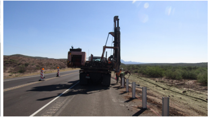
INSTALLATION OF NEW GUARD RAILS ALONG ROUTE SIX
